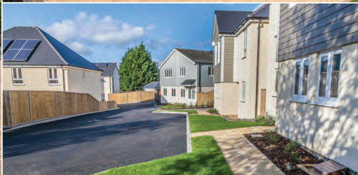
Contemporary New-Build Homes
